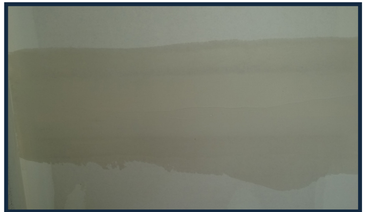
(Figure 2-29) back and forth, you will have to run this seam like a butt joint.
