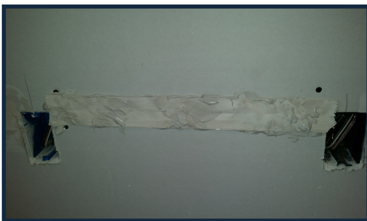
(Figure 2-14) taped first, then the flat joints, then the angle seams.
