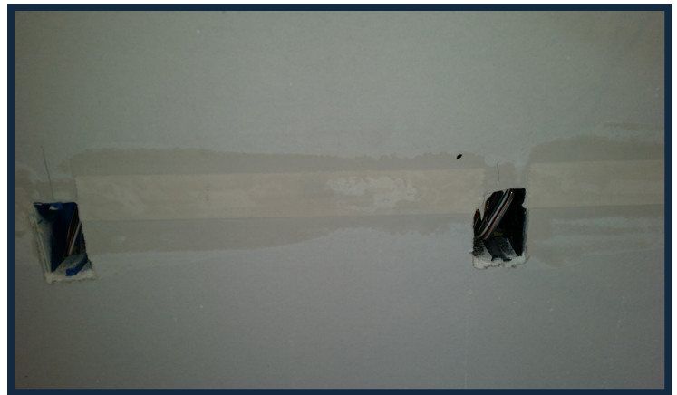
(Figure 2-15) Try to keep all of the slack out of the tape if you can, this can be done by applying some pressure on the tape while stretching it out. The wiping down process will be easier if the tape is tighter.
